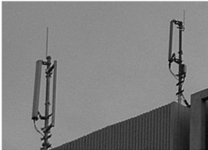
Figure 20.11 Reversed downtilting. This example is from Prague where this type of solution can often be observed.
