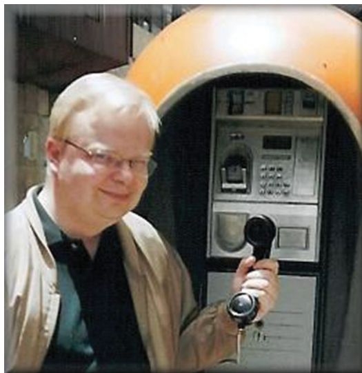
Figure 2.6 An example of the work of UNDP in the modernization of the public telephony infrastructure and equipment in Honduras. Old cabinets are investigated in Tegucigalpa, Honduras.
