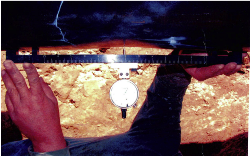
Figure 2-1-3 Measuring the depth of a dent.
