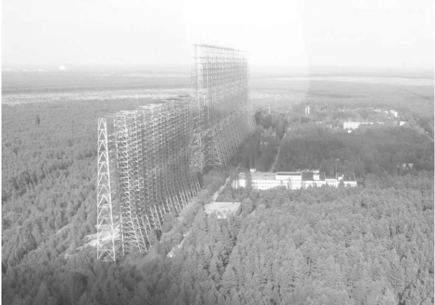
Figure 2. The over-the-horizon antennas of the radar complex at Chernobyl-2.
