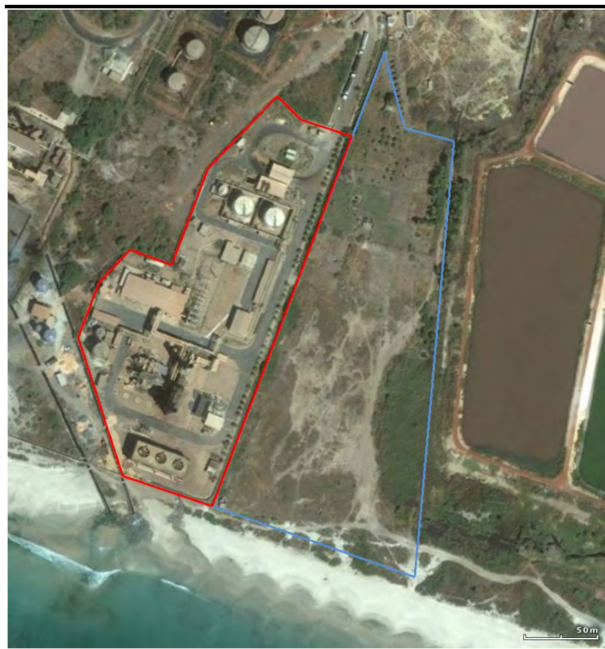
Figure 3.2 Installation site for the new equipment
