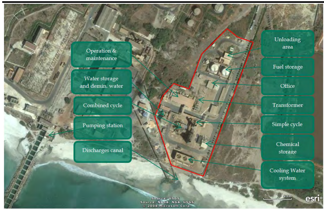
Figure 3.3 Main facilities at the existing thermal power plant
